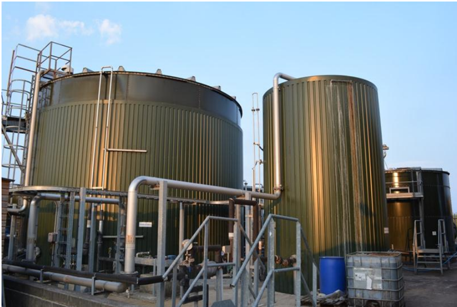
Figure 7. The Andigestion 300 m 3 digestion facility at Waterbeach
