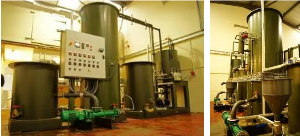
(a) Front view showing (L – R) RWBT, control panel, primary digester, storage tank and gas holder (b) Rear view
